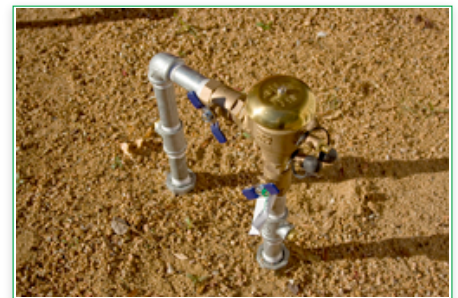
PVB - Pressure Vacuum Assembly
