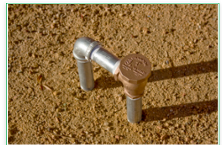
AVB - Atmospheric Vacuum Breaker
