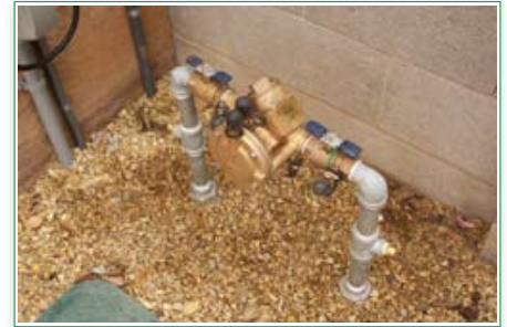
RPA - Reduced Pressure Assembly
